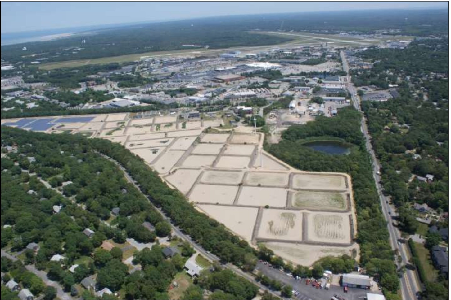
Filtration Beds – Water Pollution Control Facility
